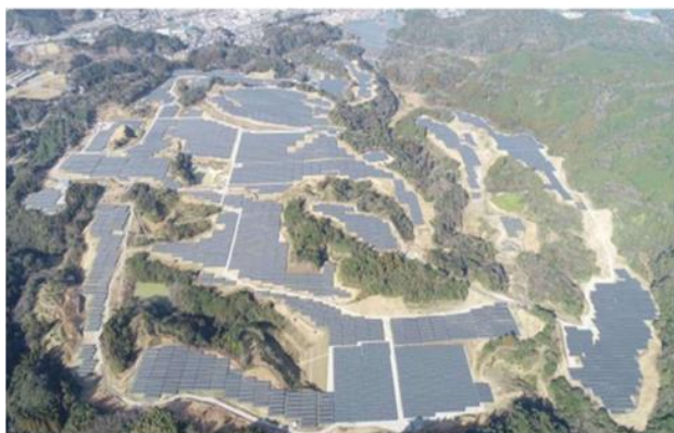
(Photo) Nobeoka-Kadogawa Mega Solar Park
