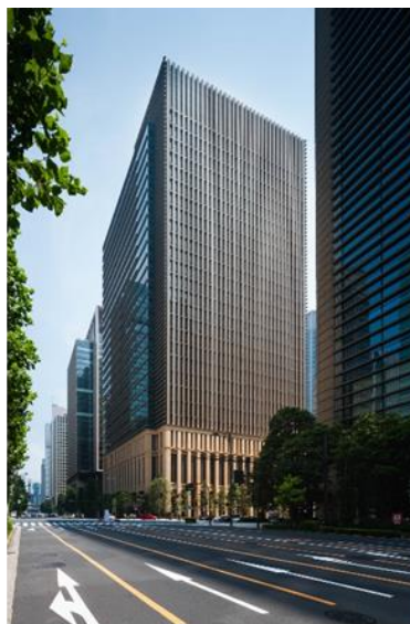
(Photo) East Tower of Sumitomo Mitsui Banking Corporation
